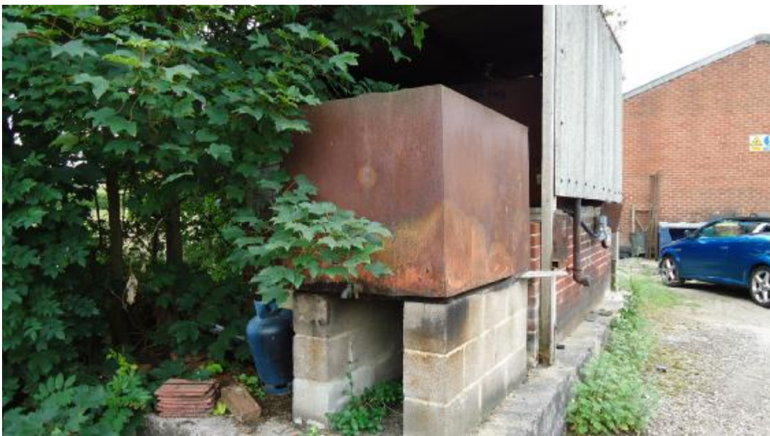
ASTs adjacent to the vehicle repair works
