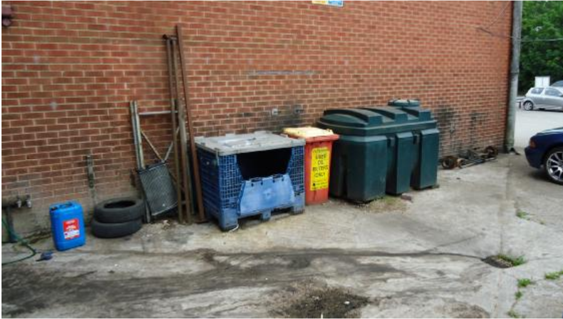
AST, old oil filter bin and other items including evidence of potential contamination migrating into the drainage system.
